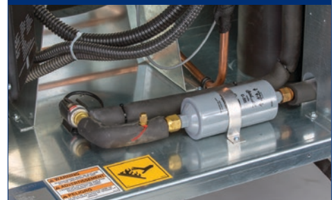
ELECTRONIC SUBCOOLING VALVE
