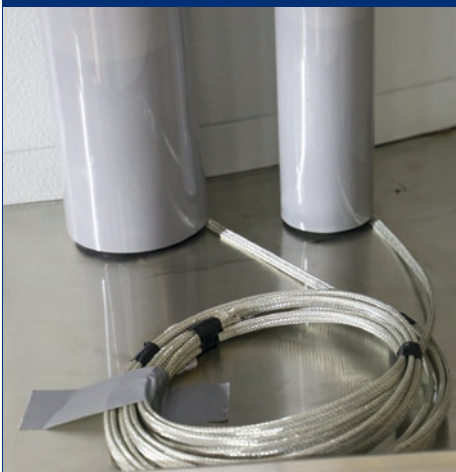
HEAT TAPE ON VENT AND CIP LINE
