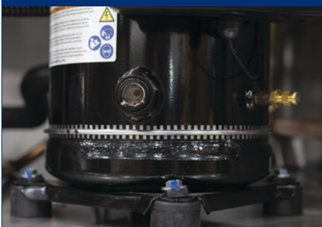
OIL SIGHT GLASS, DRAIN PORT, AND CRANKCASE HEATER
