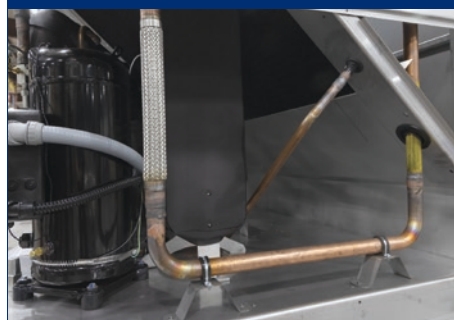
DISCHARGE LINE HEAT RECOVERY CONNECTION TUBE
