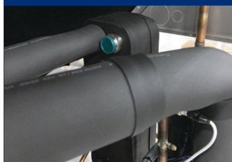
BRAZED-PLATE HEAT EXCHANGER GLYCOL PORTS
