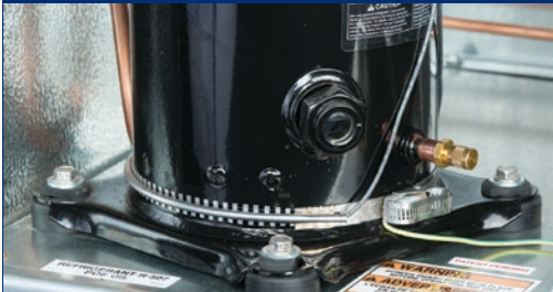
OIL SIGHT GLASS, DRAIN PORT, AND CRANKCASE HEATER
