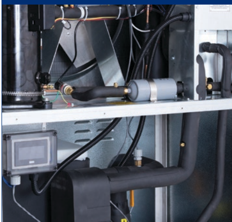
PRE-PACKAGED CHILLER REFRIGERATION PIPING
