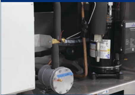
REPLACEABLE SCROLL COMPRESSOR, SERVICE VALVE, AND CORE FILTER DRIER
