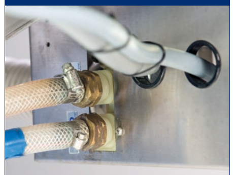
HOT AND COLD WATER SOLENOIDS
